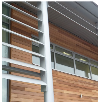
Visitor centre / offices exterior
